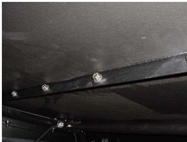
Fig. 8.4 (view of bolts between roof halves)
